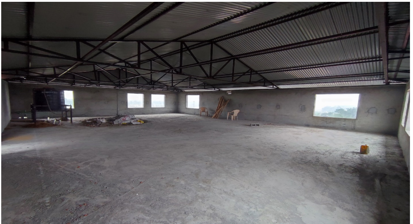
Pic 6: Hall prepared using hollow block on 4 th Floor, Snake Bite Treatment Block
